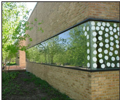
Chicago Botanic Garden Regenstein Center. The long window on the left shows the clear reflection of sky and trees before the window was treated. This is very typical of the type of reflection that birds mistake for a continuation of the outdoors. The window on the right has the temporary circular shading solution. After both windows were fully treated, bird collisions declined dramatically and immediately. Photo Joan Vatz
